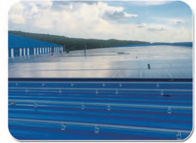
4 MW SFS-PR-01 Tin Roof Clamp Racking (Vietnam)
