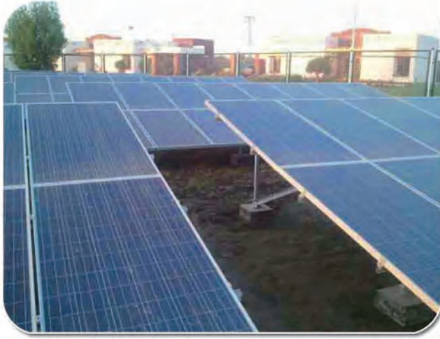
1.4MW SFS-GM-01 Concrete Base Mount System(Kazakhstan)
