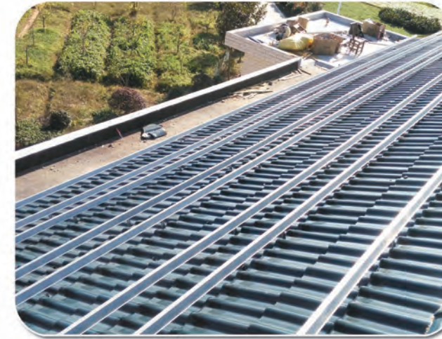
500KW SFS-PR-01 Tile Roof Mount(Australia)
