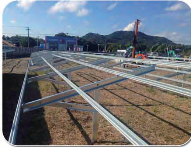
3.5MW SFS-GM-04 Pile Ground Mount Structure(Japan)
