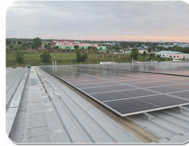
2MW SFS-PR-01 Tin roof solar mount (Vietnam)
